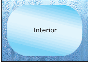
Condensation on the interior face of an IGU.
